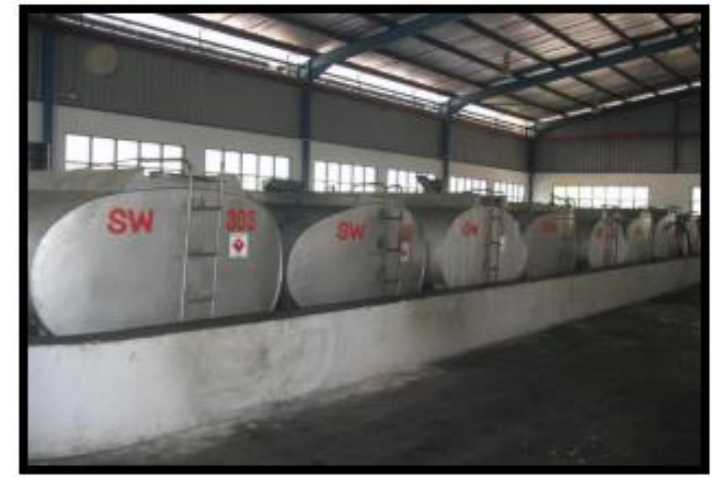
Figure 4: Storage tanks for waste oil. The capacity of the containment should be 110% of the largest container stored.
